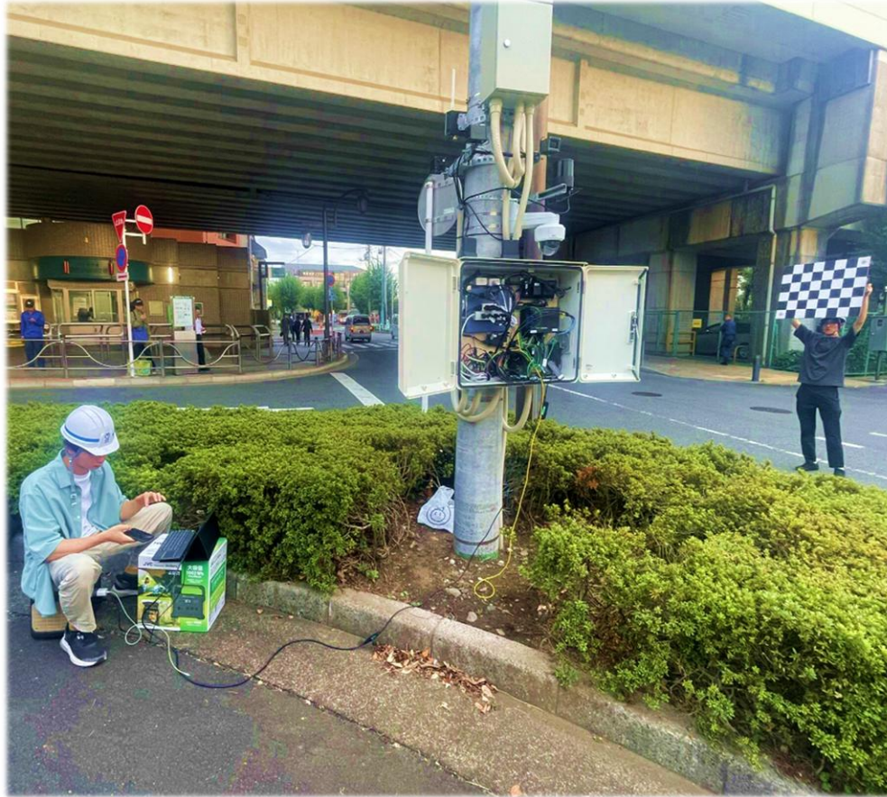
Smart pole deployment & calibration (roadside infrastructure)
