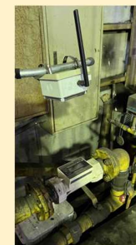
Gas meter and camera view Camera captures gas usage and AI analysis
