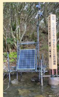
Surveillance cameras on the lakeshore & Solar panels and batteries
